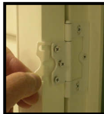
Insert hinge spacer.
