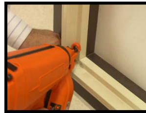
Only secure one nail into the bottom left frame.
